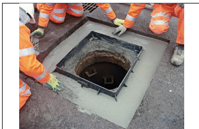
Figure 1 Preparation of substrate ready for the backfill
